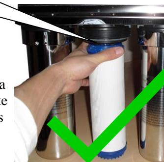
After replacing the inner filter, use the special screwdriver to tighten the stainless steel cylinder. Switch on the inlet, open drinking water faucet, and then shut off the faucet. Use a piece of paper napkin to wipe the joints to make sure the napkin does not get wet so that there is no leaking. If there is a leaking, repeat STEP 1 and STEP 2, and then tighten the cylinder.
